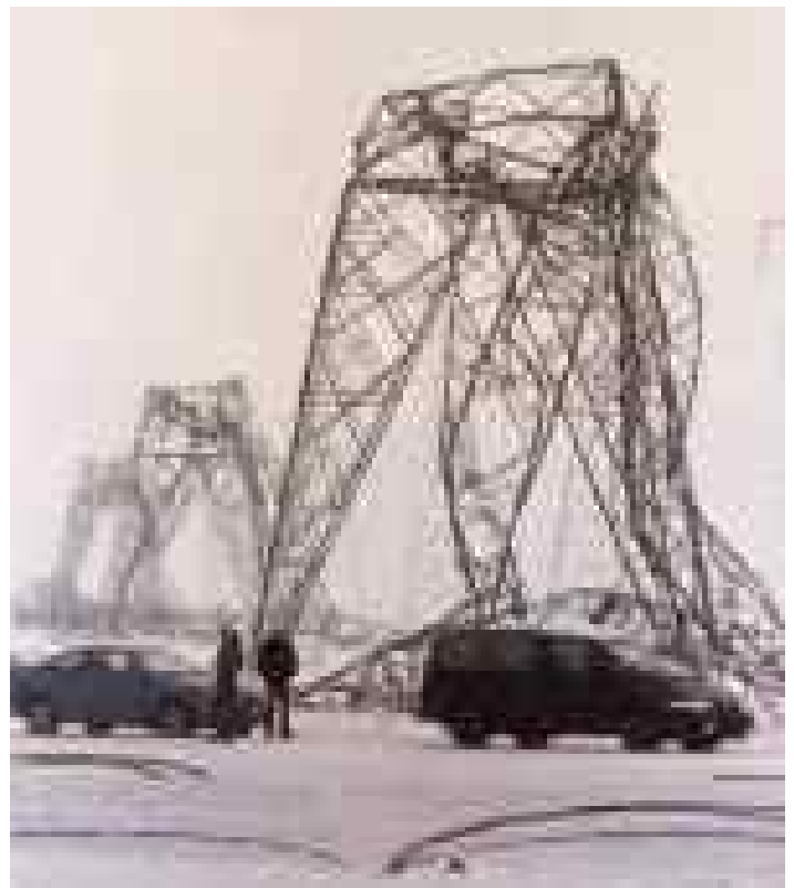
Figure 1 Dramatic evidence of the power of ice on the power industry. One hundred foot tall towers carrying power lines are seen here bent like blades of grass in the aftermath of the 1998 ice storm that hit southeastern Canada and the Northeastern US.
